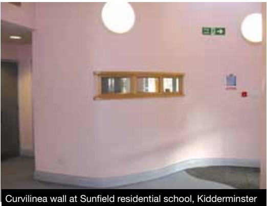
Curvilinear wall at Sunfield residential school, Kidderminster
