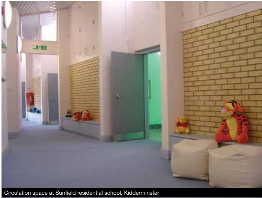
Circulation space at Sunfield residential school, Kidderminster
